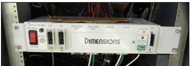
Bypass Switch installs in DC 336 "stretch" cabinet
